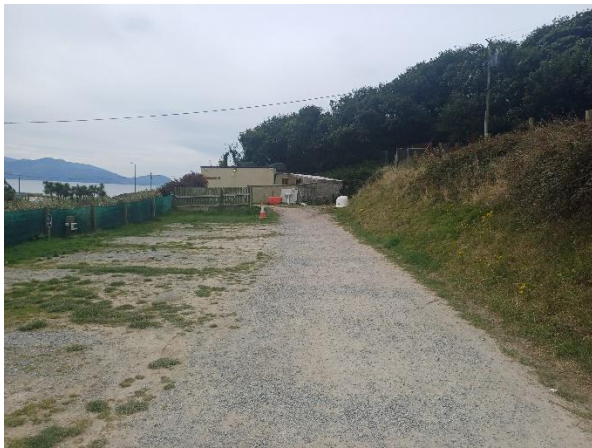
View to west toilet/shower block from within campsite
